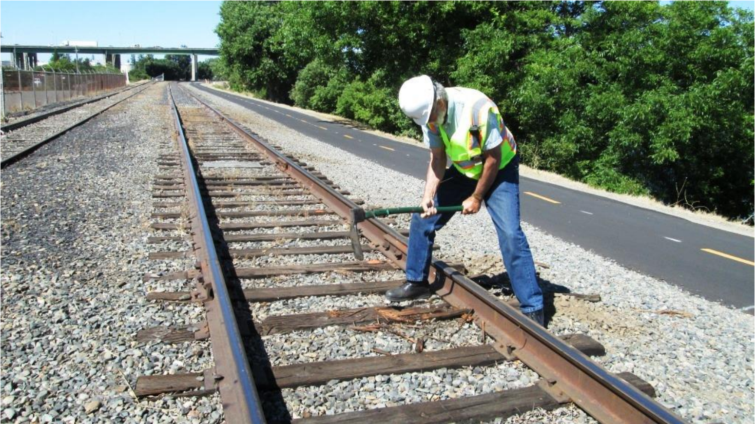
Alan uses an adz to shave-off high spots on plate-cut ties that could get caught on the base of the rail when pulled
