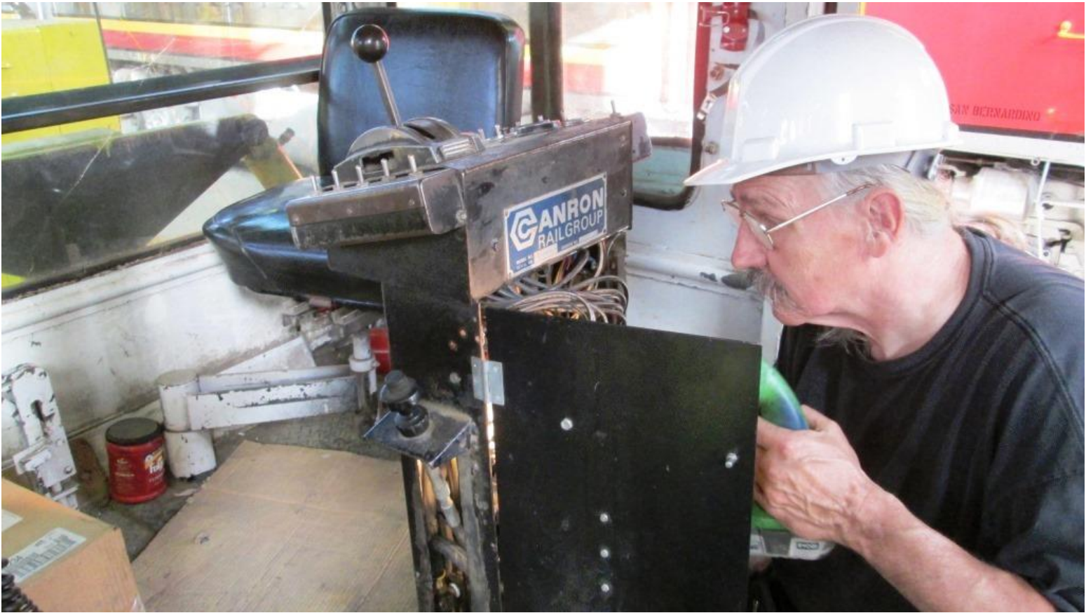
Fred traces air-lines in the control stand of the regulator
