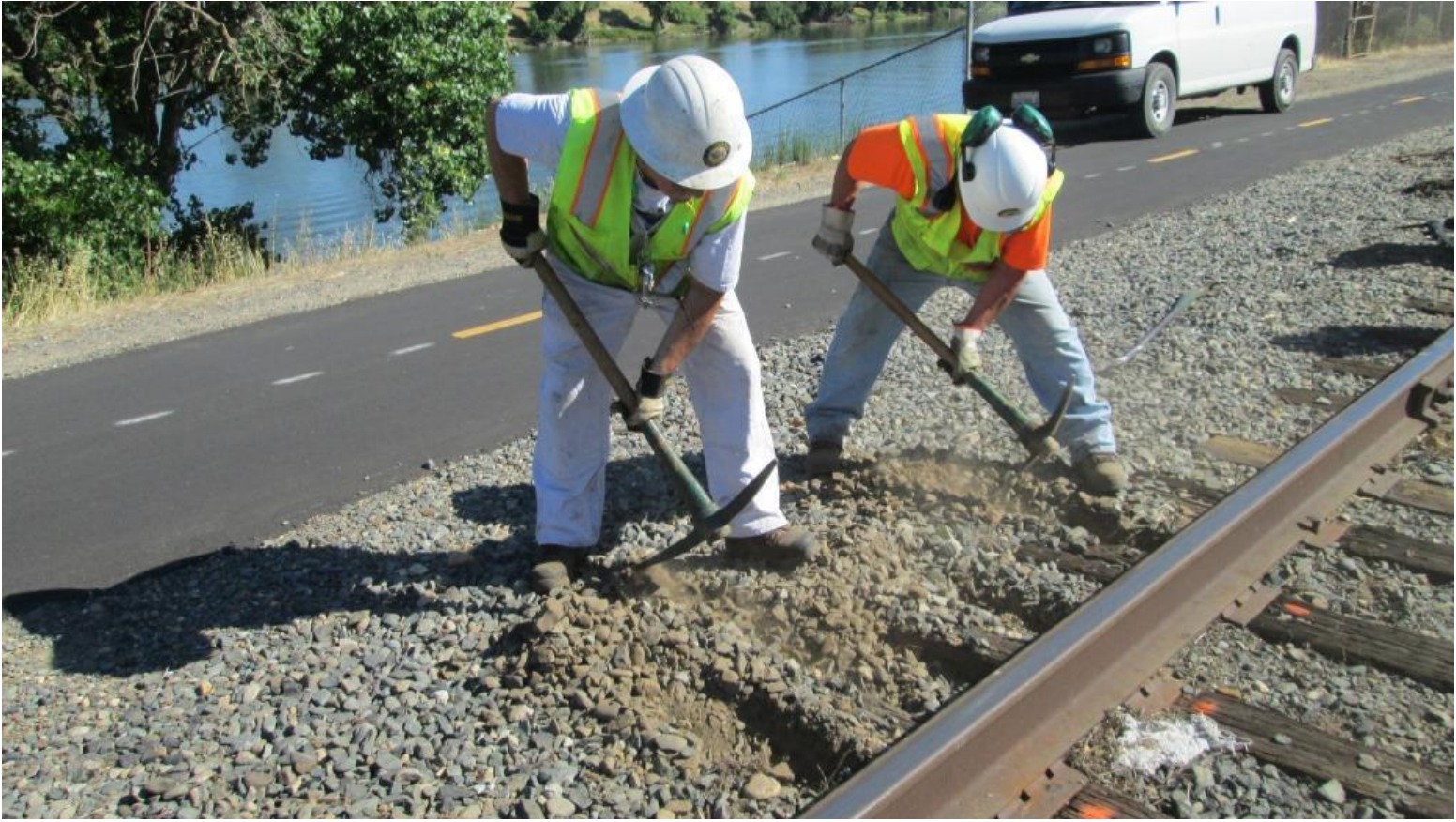
In a team effort, Mike H. and Joe clear away rock from the ends of ties marked for removal
