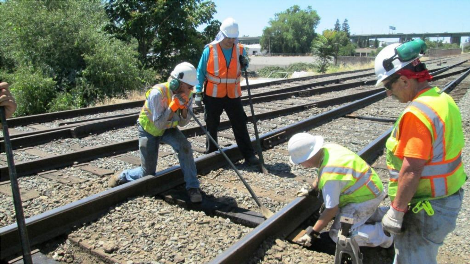
Steve nips-up the rail so that Mike H. can shimmy a tie-plate between it and the tie
