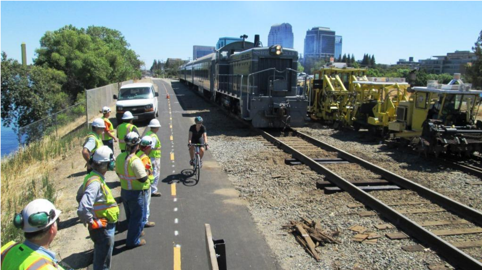
Quite the convergence: the MOW Team stands back as a bicyclist and the train pass through our work limits
