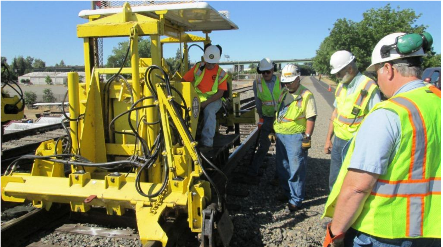
Joe gets a captive audience when he starts pulling ties with the Jackson 125 tie-exchanger
