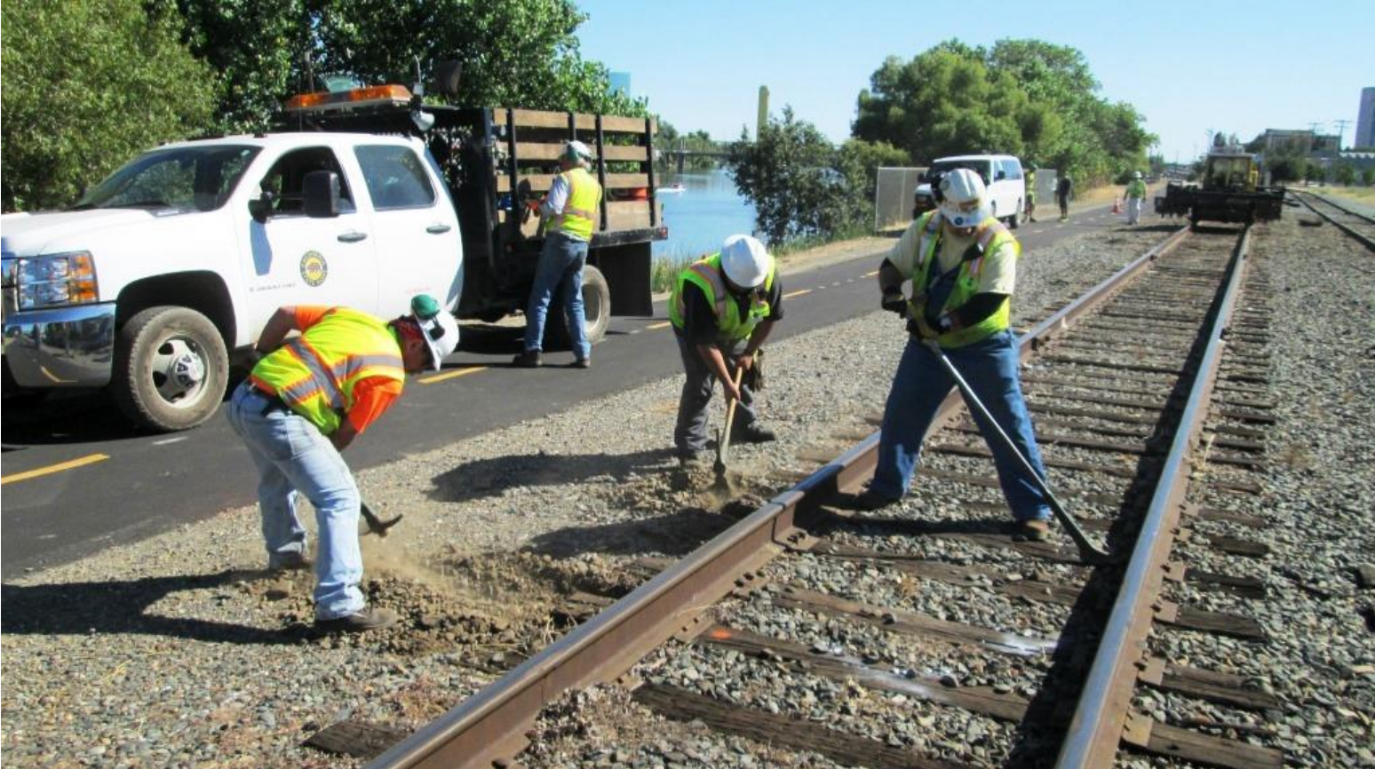
At Clunie, Joe and Anthony dig around tie-ends while Mike F. pulls spikes
