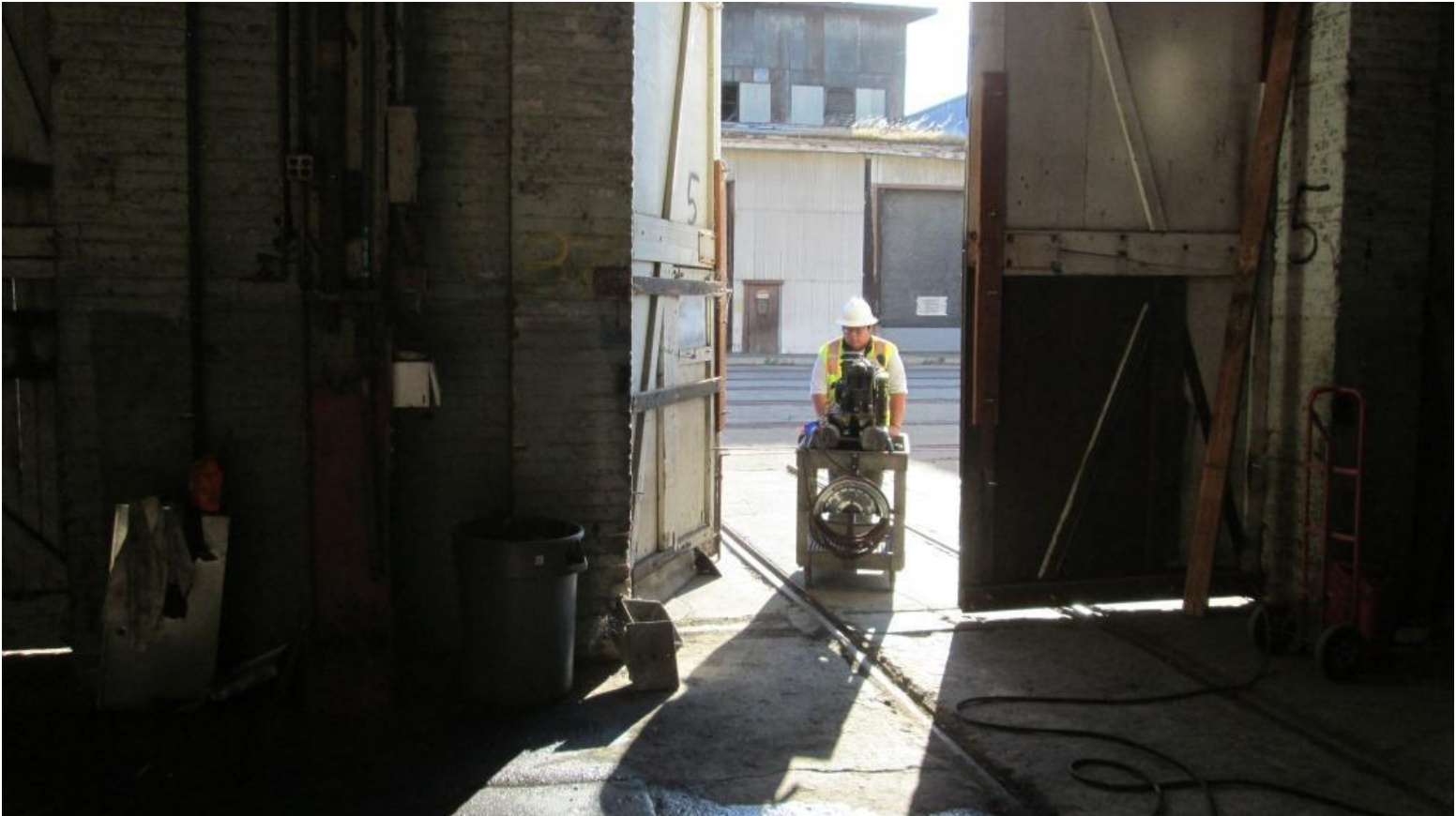
Anthony brings the air-compressor on a cart into the Erecting Shop
