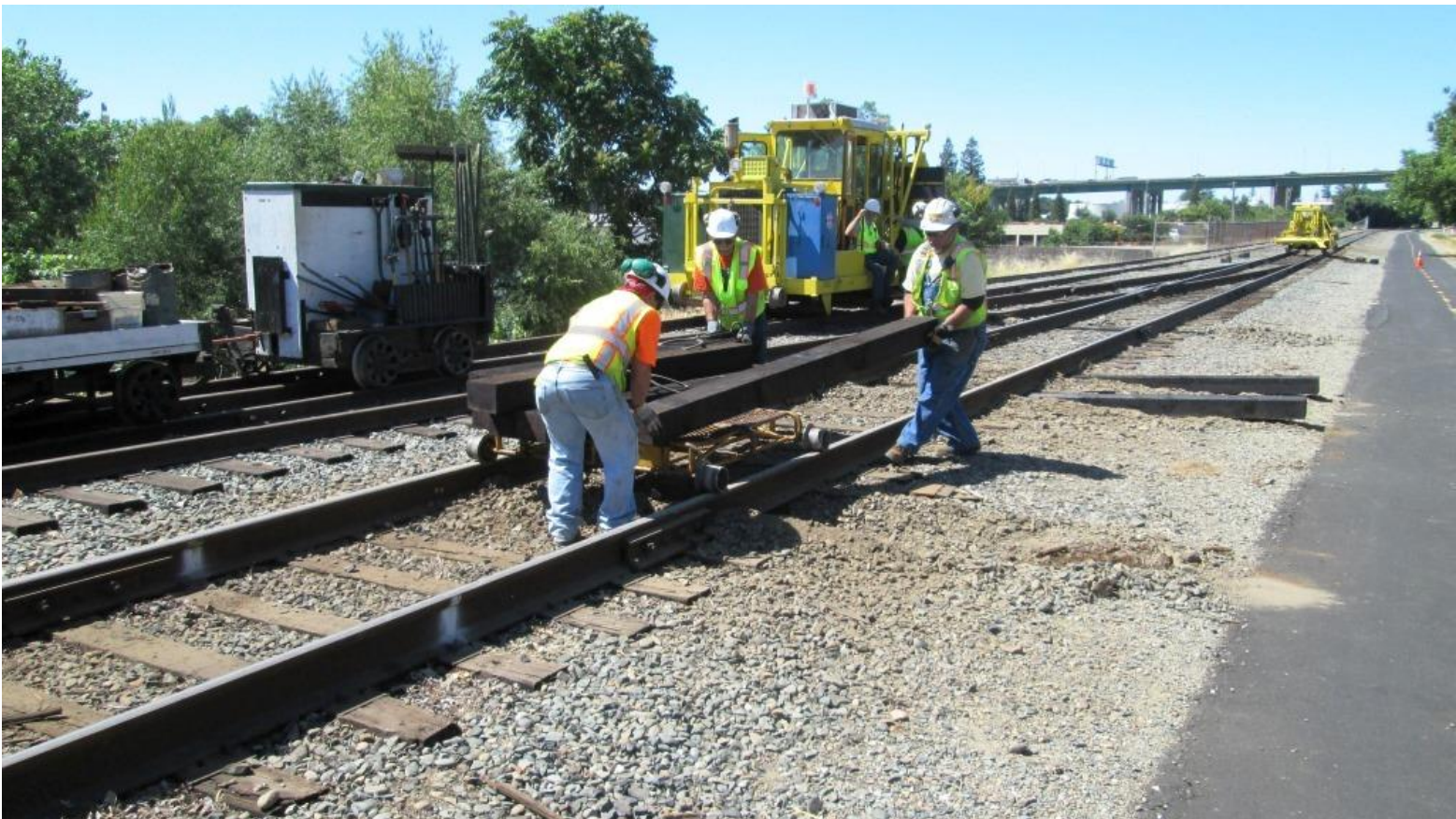
New ties are set into the empty tie-cribs for the scarifier-inserter to pull into place
