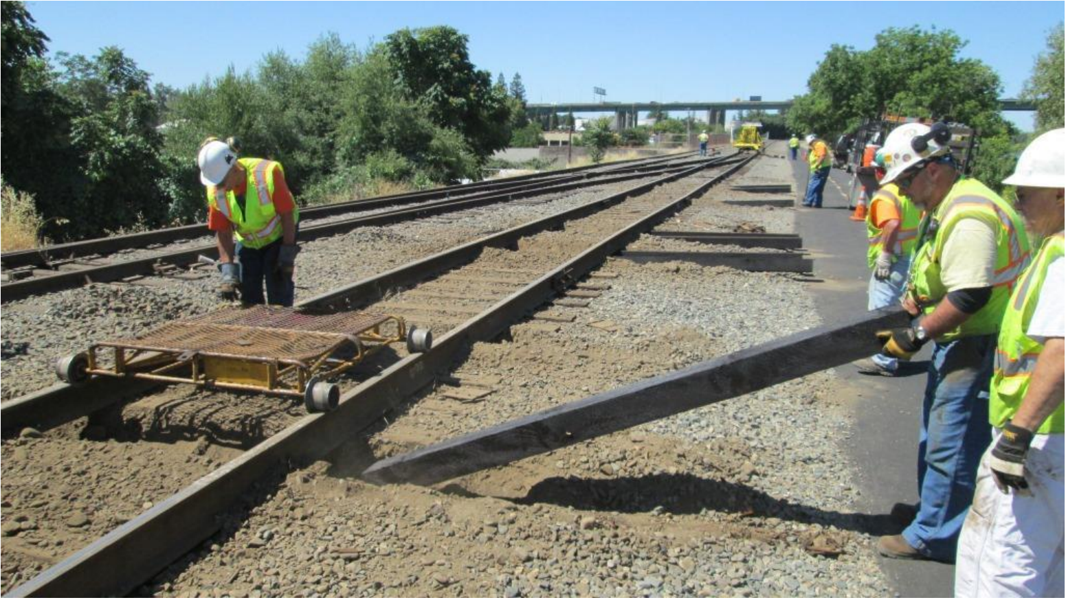
Mike F. lines a tie up for insertion
