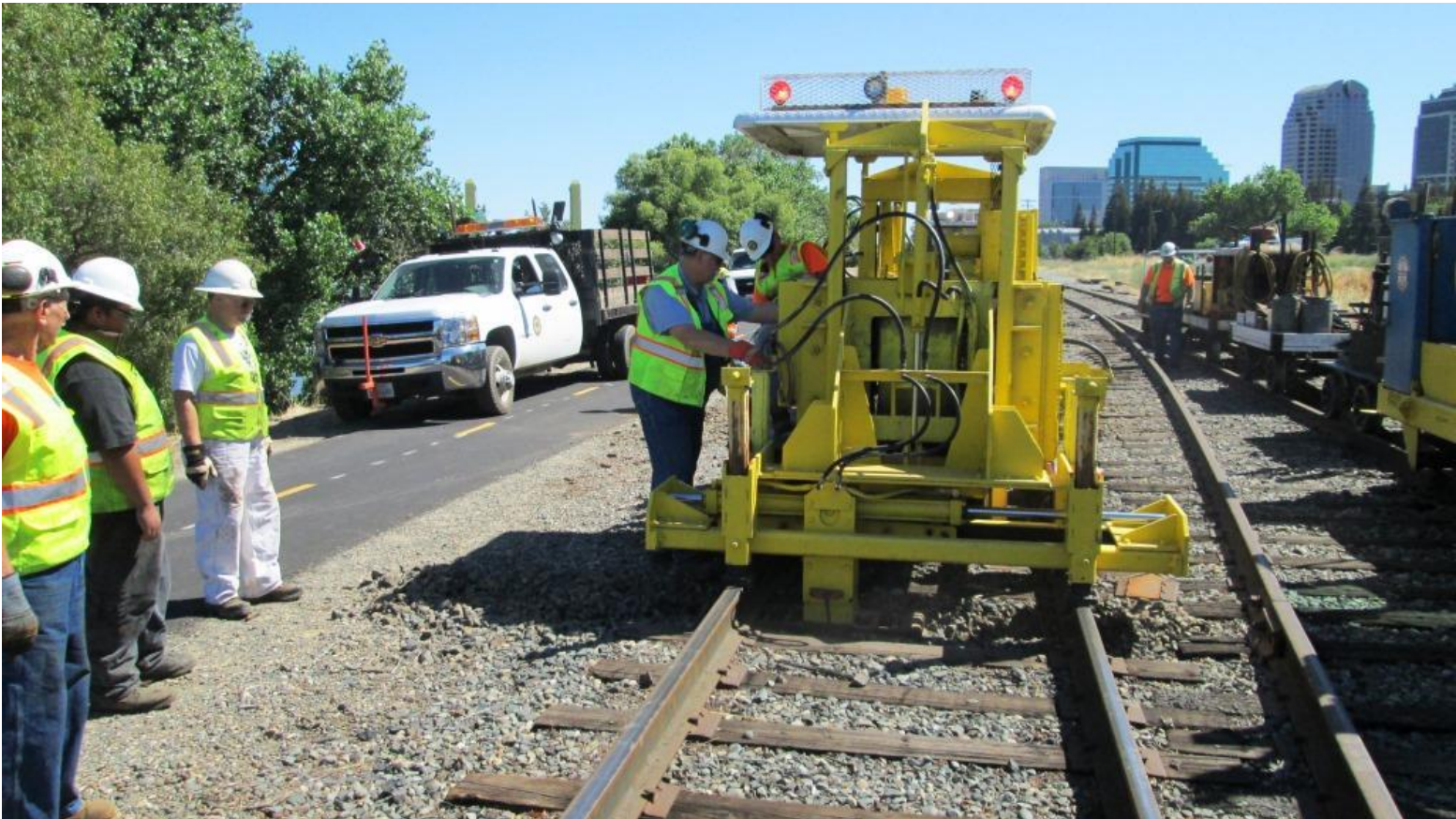
Chris shows Joe how to use the scarifier function on the 125 which works perfectly for tight areas where two tracks converge
