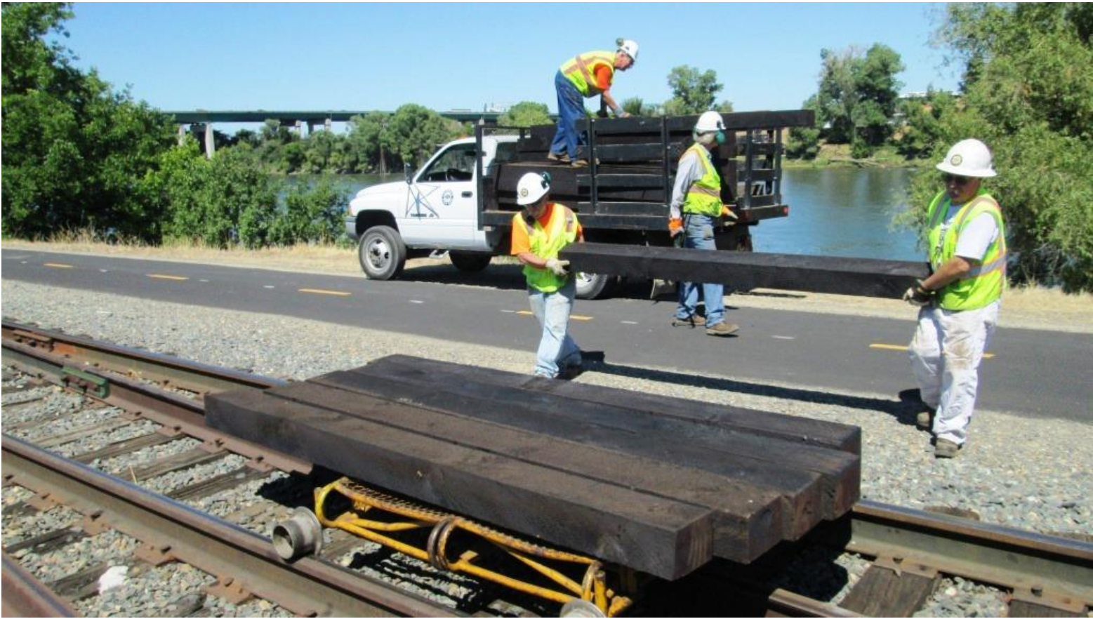
Clem drops new ties from the truck as Joe, Mike H., and Steve load them onto the Nolan track cart for distribution
