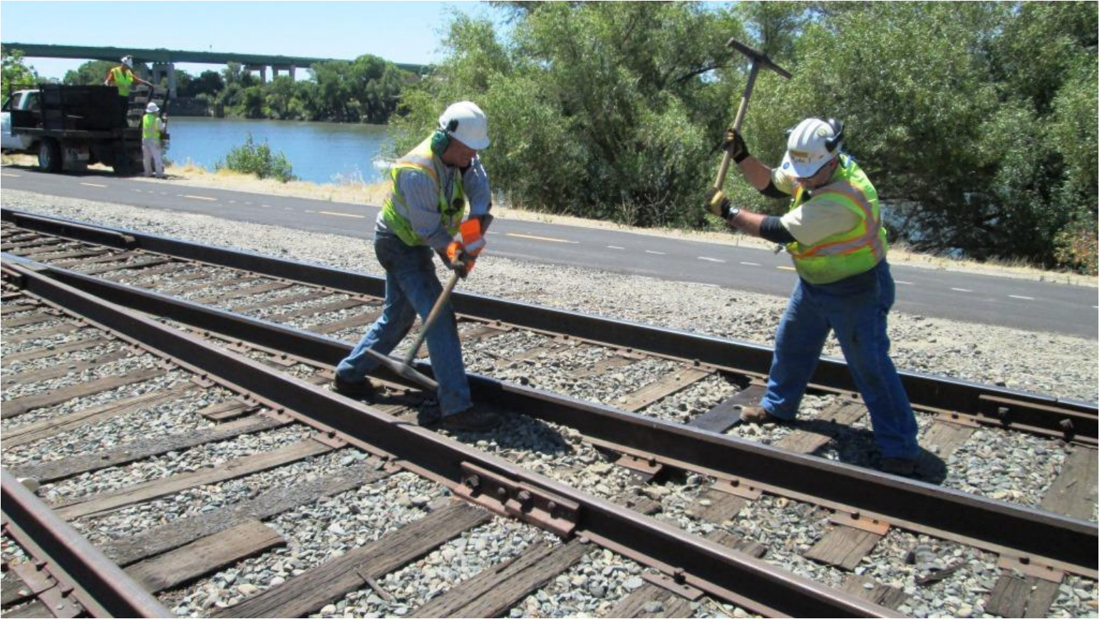
Steve and Mike F. interpret good ol' fashion track-gang railroading with a tandem spike-driving demonstration
