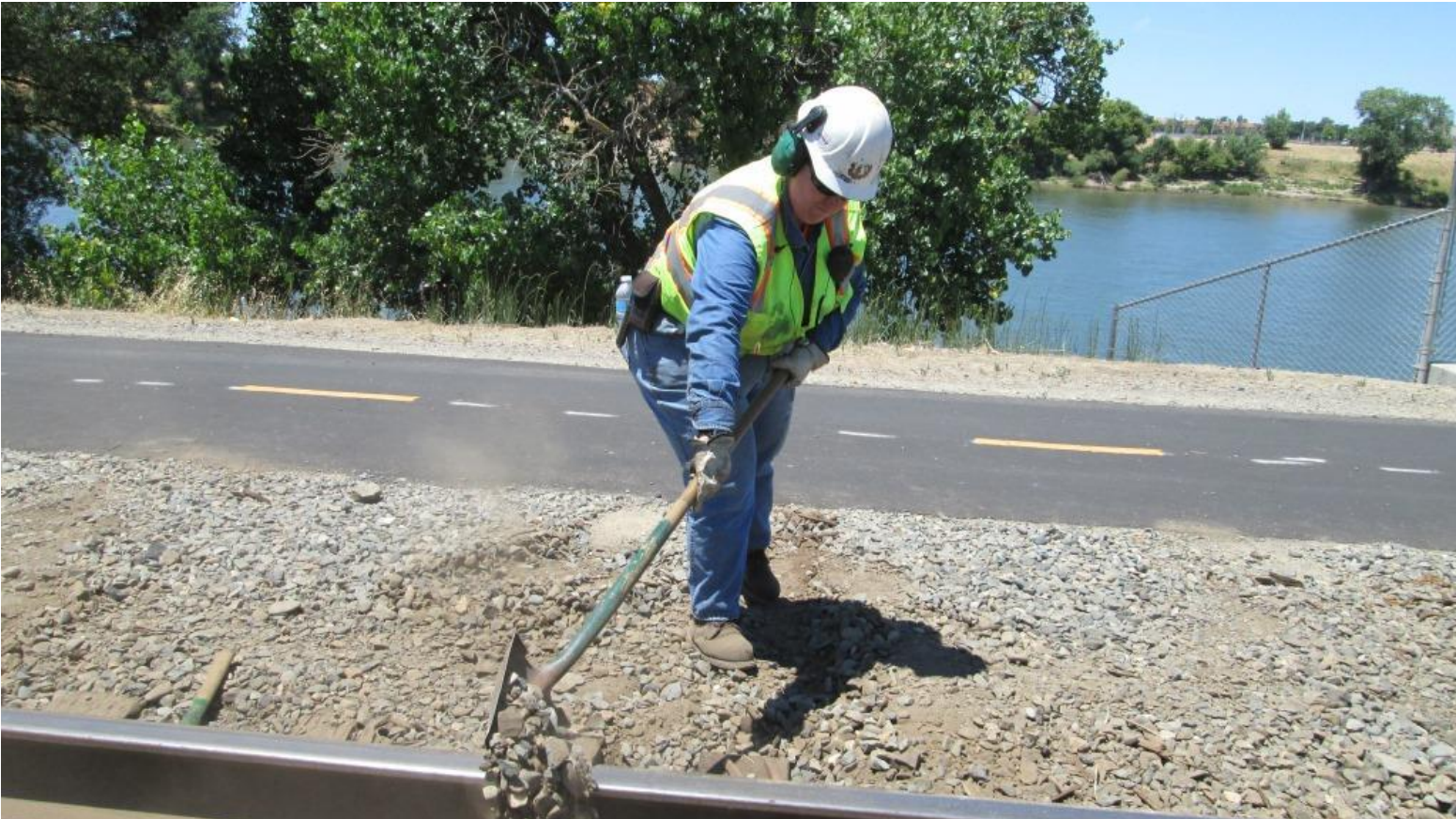
Heather fills in around the new ties with rock
