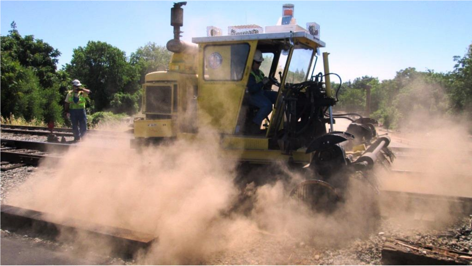
Heather kicks-up some dust as she scarifies the crib of the last tie pulled for the day
