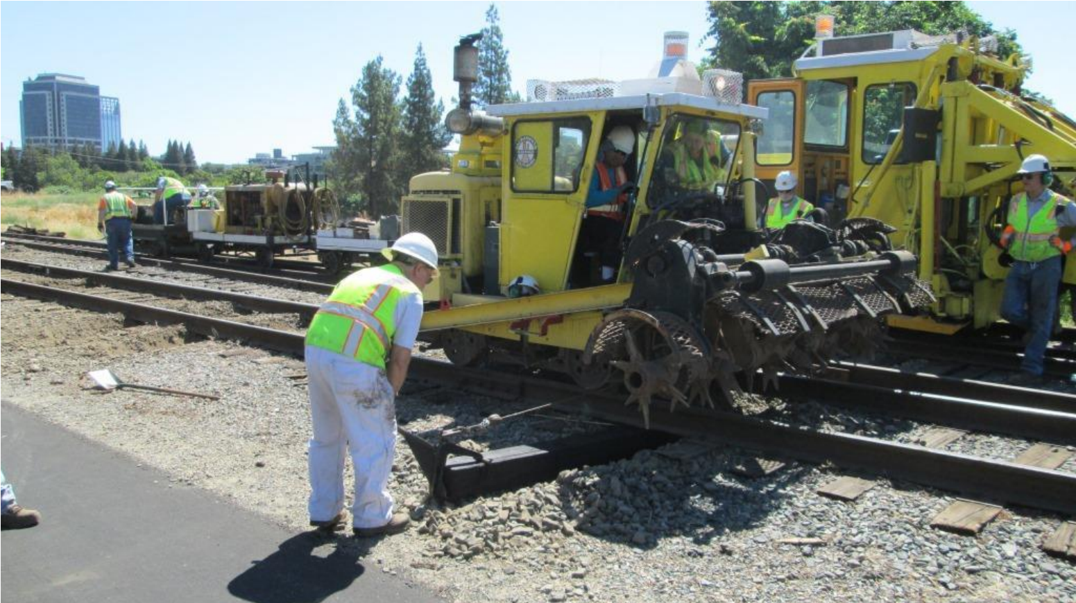
Mike H. guides a new tie into place as Jose operates the scarifier-inserter with Heather as trainer
