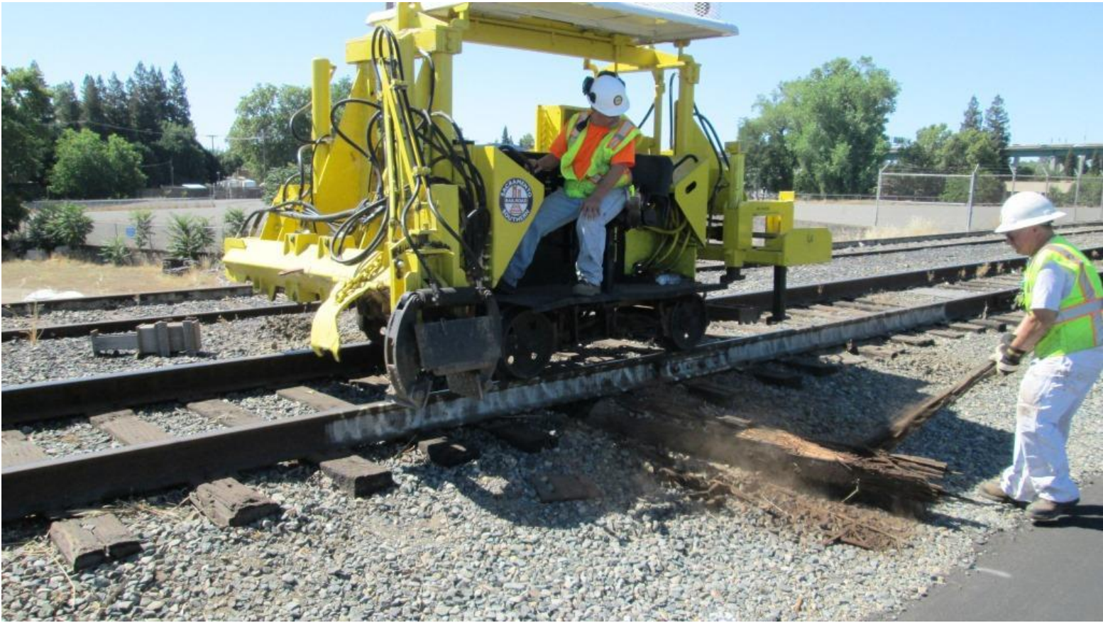
Many ties disintegrated as they were removed
