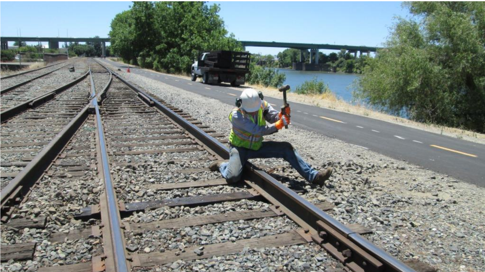
With new ties in place, Steve sets spikes
