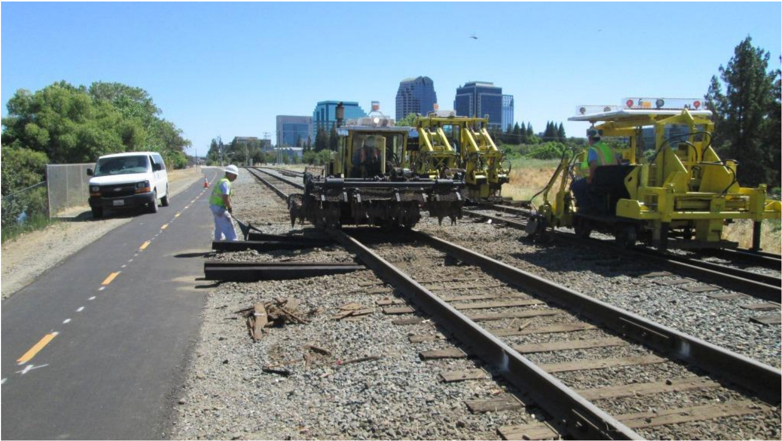
Mike H. and Jose pull in the remaining ties
